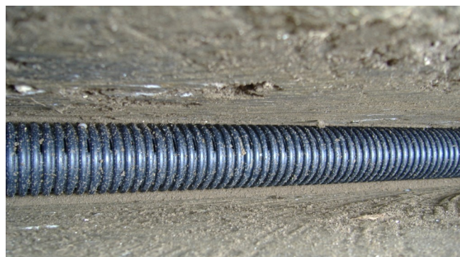
80mm pipe fits snugly in a 97mm trench
