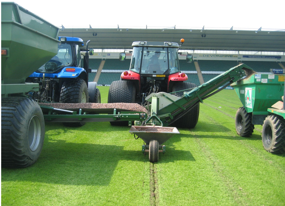
System 25 installing secondary drainage, Gravel Cart keeps hopper topped up
