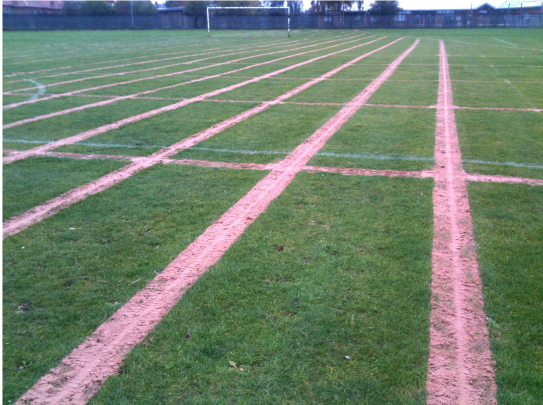
Sand Slits installed at 2 metre centres at 90 degrees to primary drainage.
