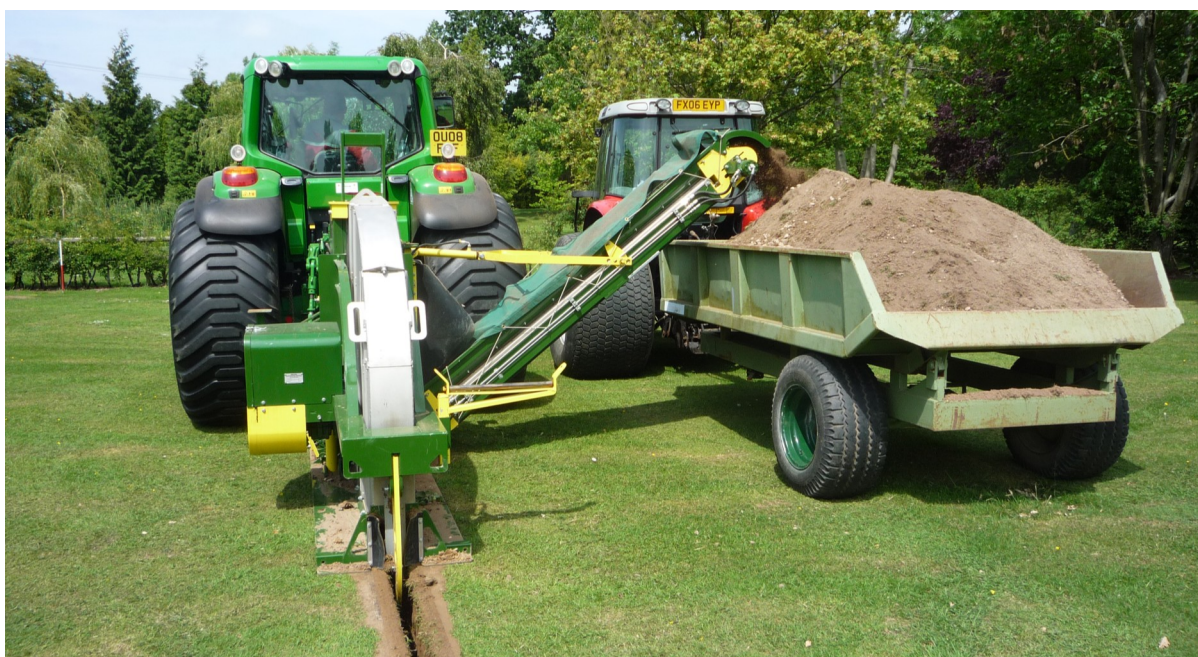
Specialist equipment ensures high work rates
